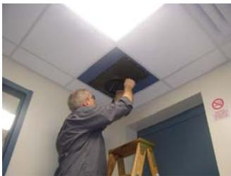
*Set up requires only a ladder to reach the ceiling, and Phillips head screwdriver.*
